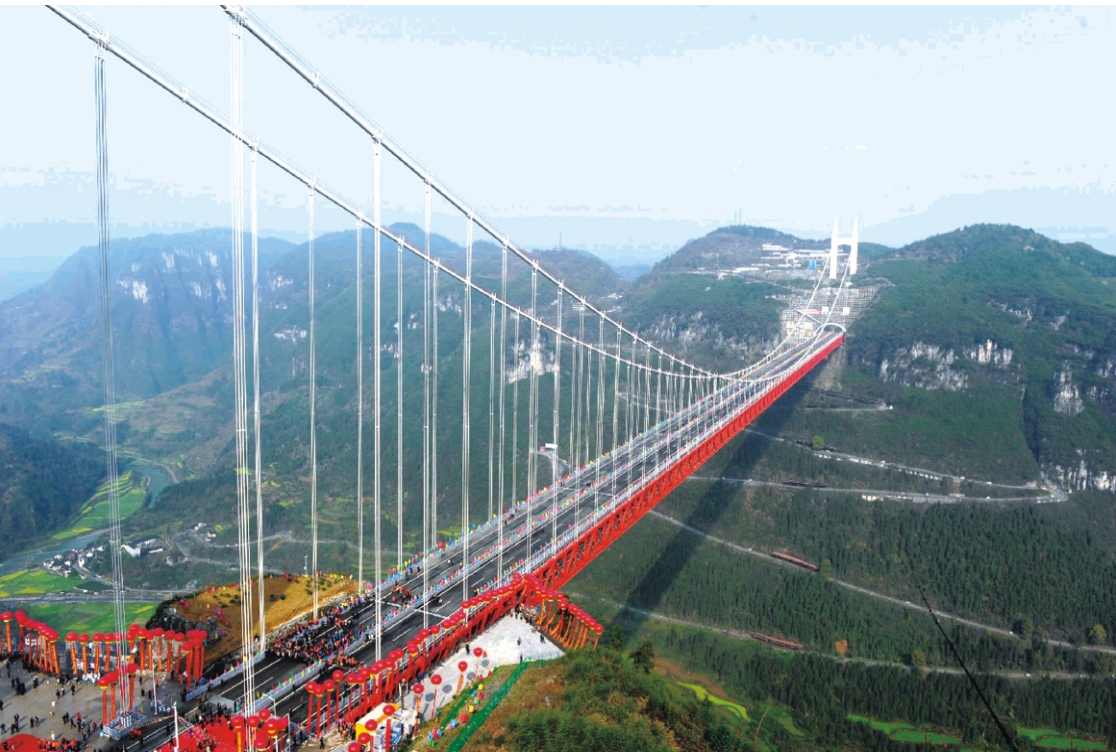
湘西矮寨大桥(带肋钢筋) Xiangxi Aizhai Suspension Bridge (Rebar)
