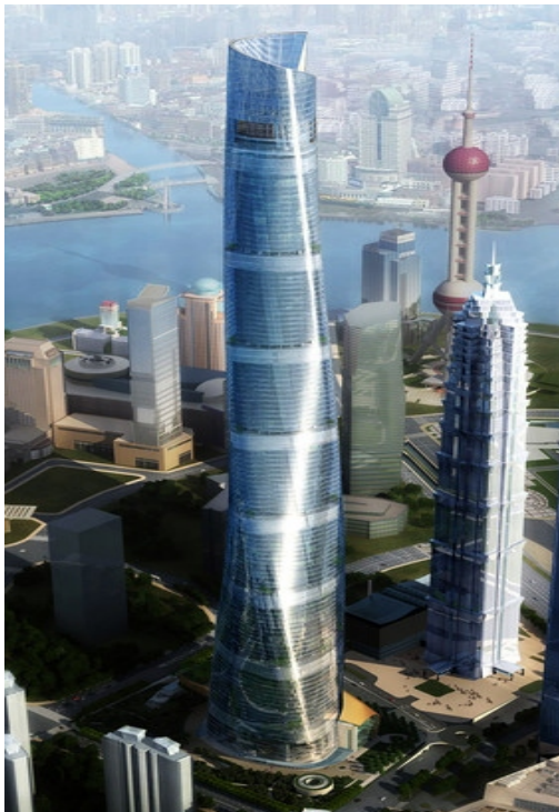
上海中心大厦(高层建筑用钢) Shanghai Tower(Steel for high-rise building)
